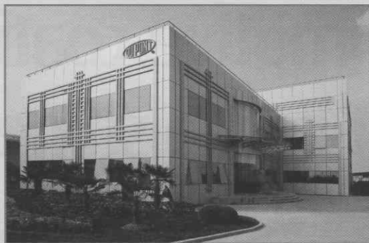
Figure 2. DuPont Coatings technical service center opened in Shanghai, China, in 2003. (Image courtesy of DuPont)
